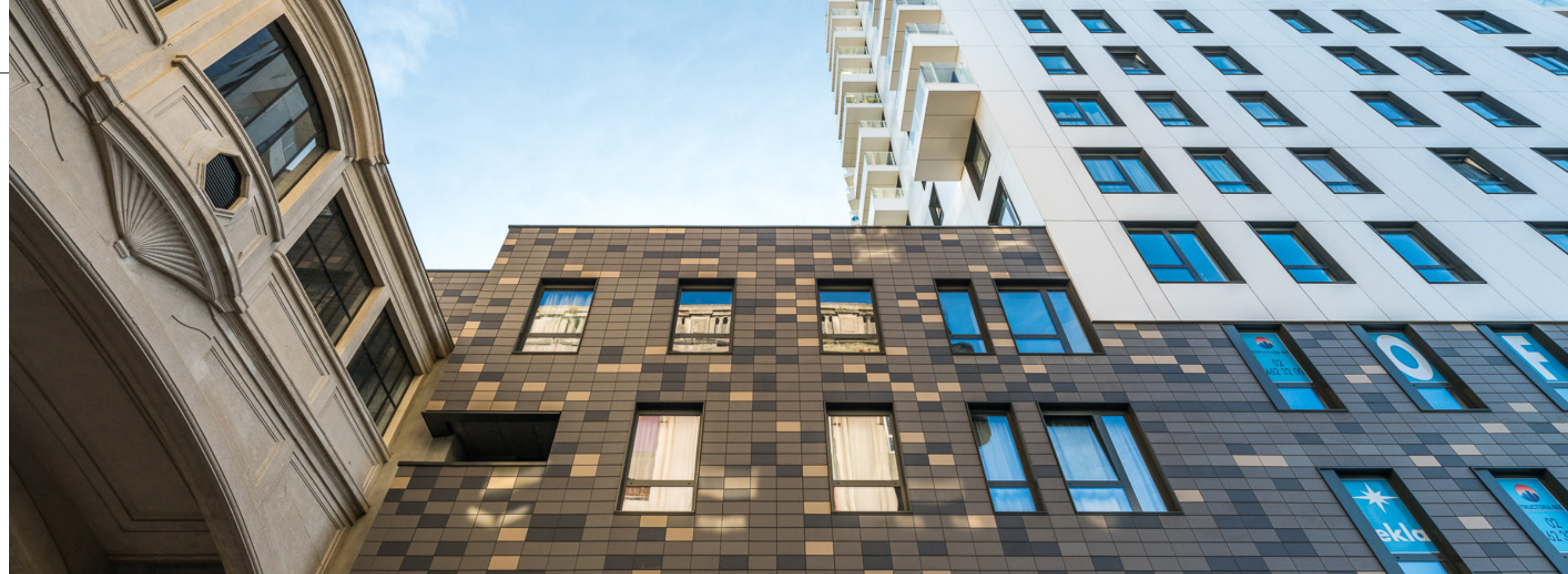
Object: Renovation in a high-rise building: Ekla tower in Brussels with Argeton® Tampa panels in various colours.
